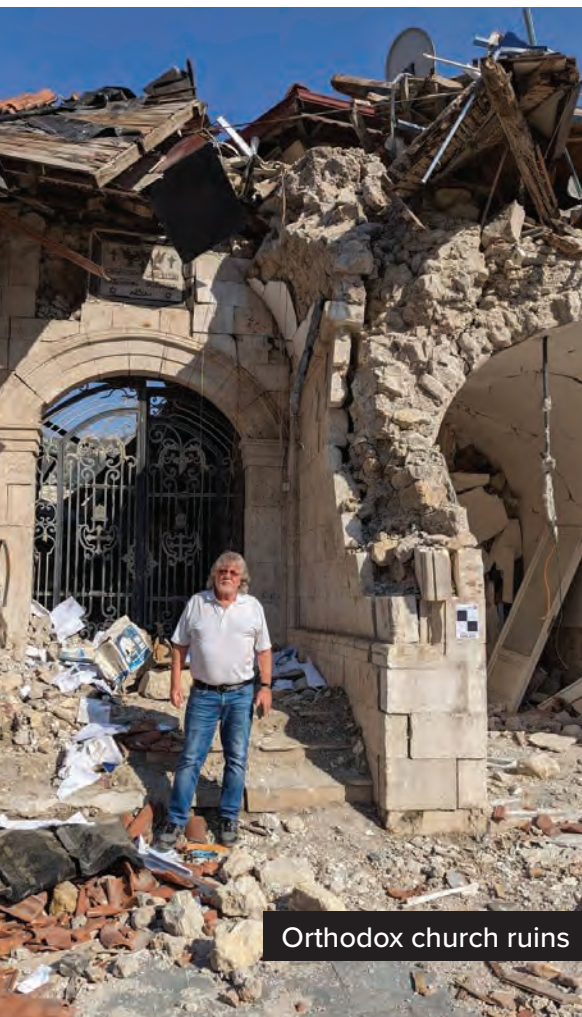
Destruction and demolition
